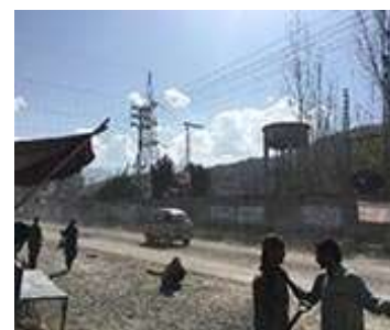
Figure 12: Images of Massive Electric pylons, Murree road-Abbottabad
