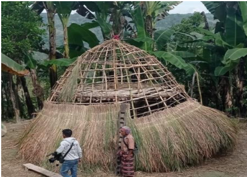
Figure 1. Ume Kebubu Construction Process
