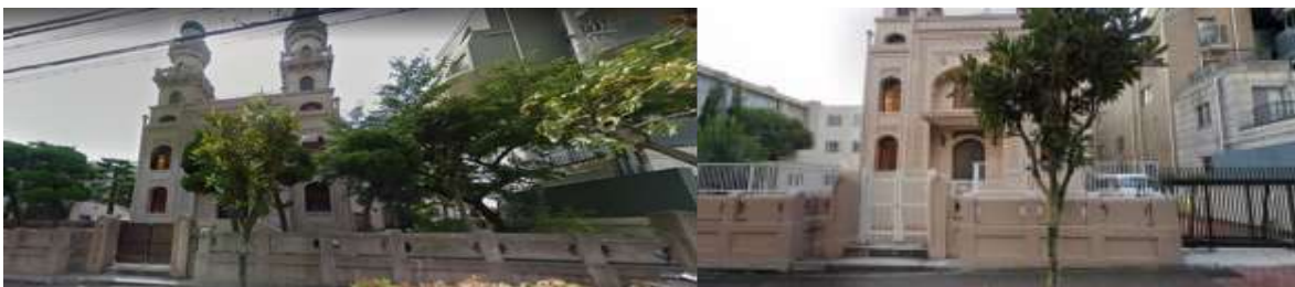
Figure 2. Building and environmental conditions of Kobe Muslim Mosque in 2016 (left) 15 and 2021 (right) 12 .
