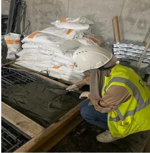
Plate (3): Casting materials for slab
