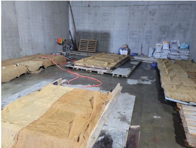
plate (5): Slabs Curing
