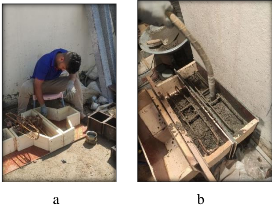
Figure (9) (a) Grease the molds, (b) electric vibrator
