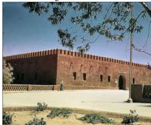
Image 17: The annex of the subsidiary circle in Tamanghast, 1960
