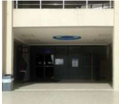
Figure 8. Inaccessible entrance COMSATS university
